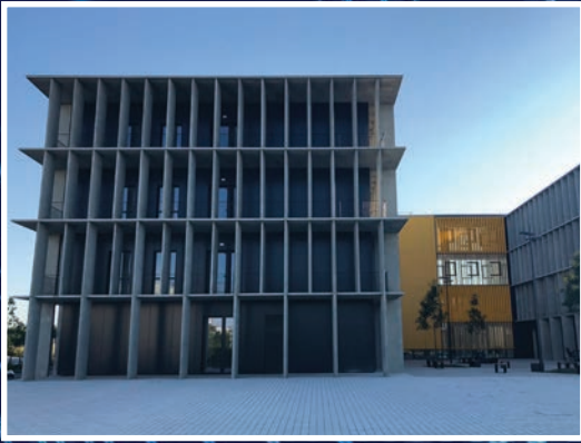
Inset: Exagan's Power Solutions Center in Toulouse, France.
